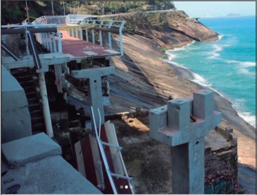
Figure 1 – Collapsed portion of the Ciclovía Tim Maia
