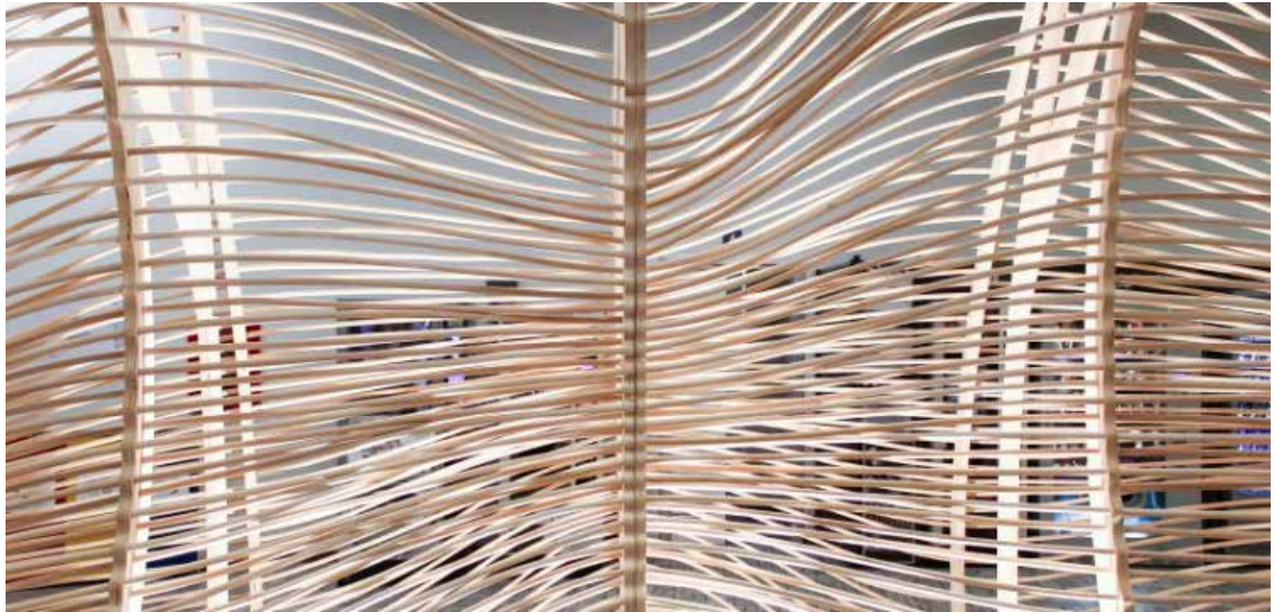
Figure 20: The variable density of rattan wefts generates a differential screening ratio along Weaving Enclosure surfaces
