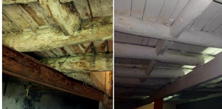
Figure 3 – Amendments currently introduced to reinforce two-story houses
