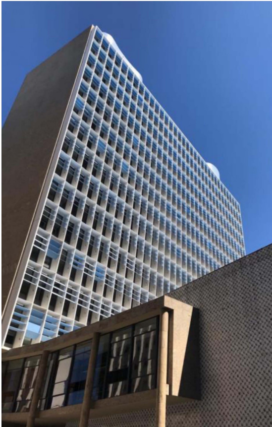
Figure 1: View of the northern facade of the MEC building (1936), Palácio Gustavo Capanema, Rio de Janeiro, with the movable horizontal shading devices. Photo: João Leal.
