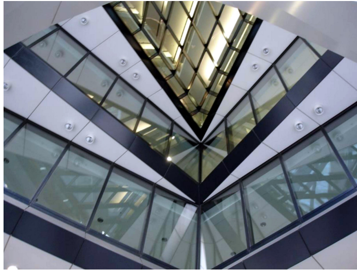
Figure 5: View from the ground floor of one of the spiralling perimetral atriums of the 30 St Mary Axe building. Photo: Érika Mitie Umakoshi.
