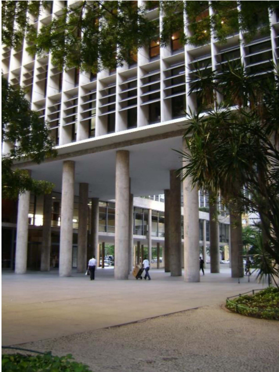
Figure 2: Ground floor of the MEC building showing the open-access shaded pedestrian area protected by the pilotis. Photo: Joana Carla Soares Gonçalves.
