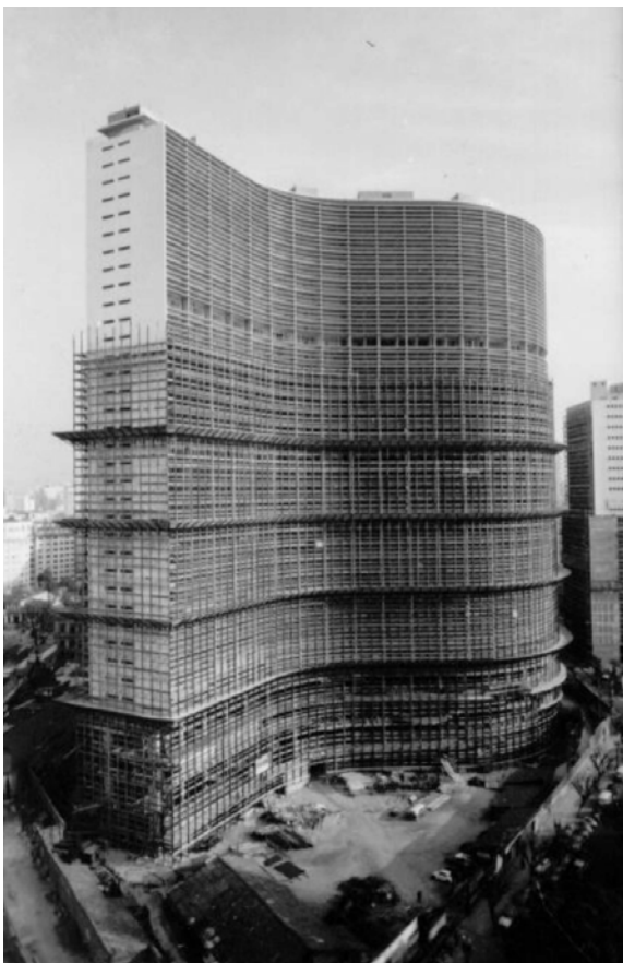
Figure 5 –Final phase of construction of the Copan Source: Copan Archive.
