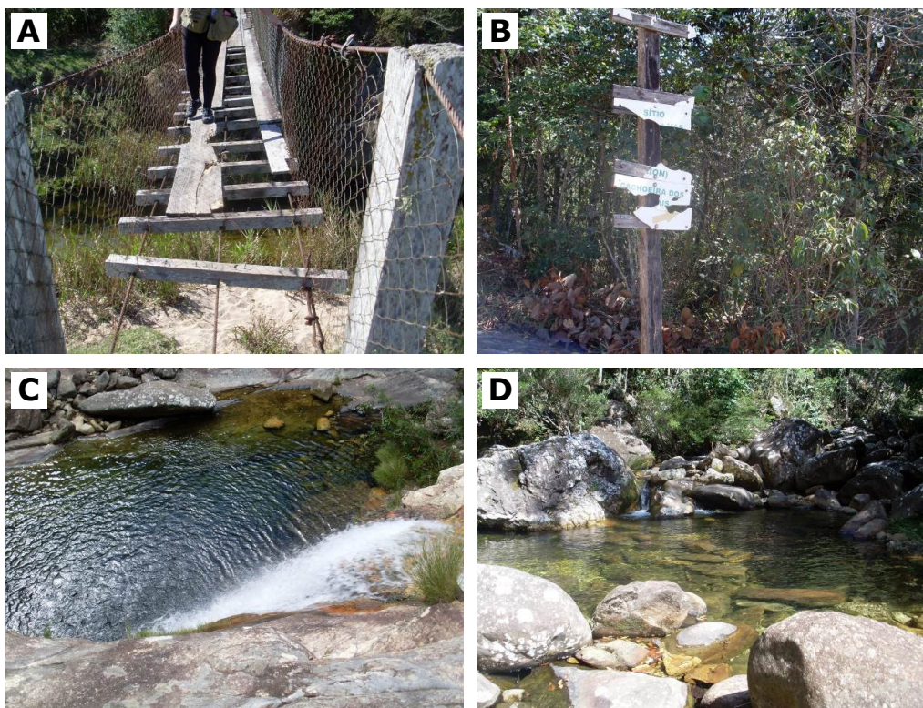
A. Wooden bridge over the River Tanque with damaged and non-existent parts; B. Damaged sign indicating Cachoeira dos Cristais and Alto das Bandeirinhas; C. First fall of Cachoeira dos Cristais; D. Wells upstream of the first fall of Cachoeira dos Cristais
